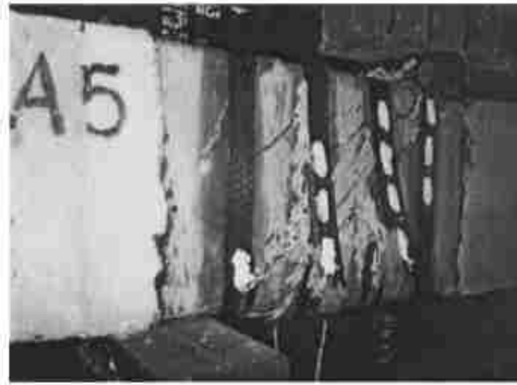
Figure 2.6. Shear Failure due to FRP Fracture (Cao et al., 2005)
